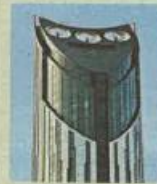
turbines at the top and 24 "sky gardens" between two glass skins around the building.
