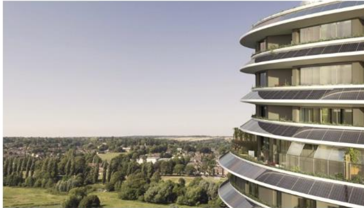
The technology will be used on future projects and the company hopes that other developers will follow in striving for carbon neutral projects
